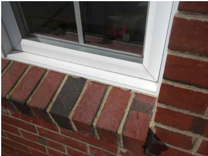
Window caulking is exhibiting cracking and separating from brick
