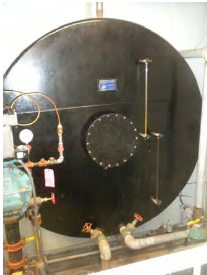
One of two large (2,500 gallon) water storage tanks
