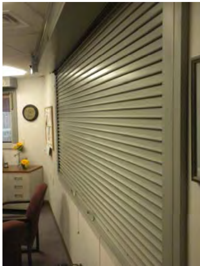
View of the fire curtain at the management office
