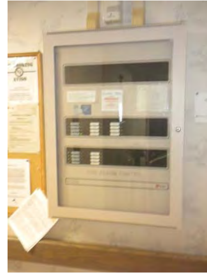
The fire alarm control panel
