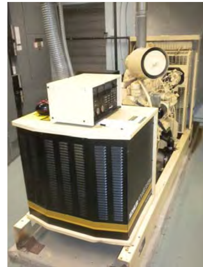
The 125 kW diesel fueled generator
