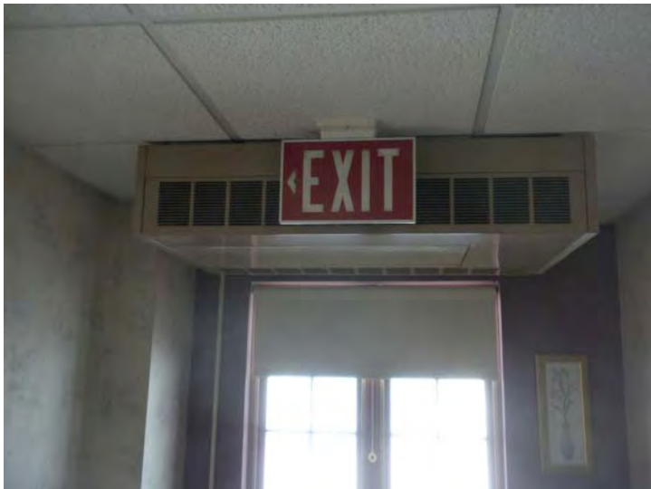
Example of the suspended space heater
