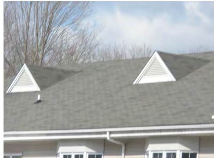
View of the composite shingle roof covering
