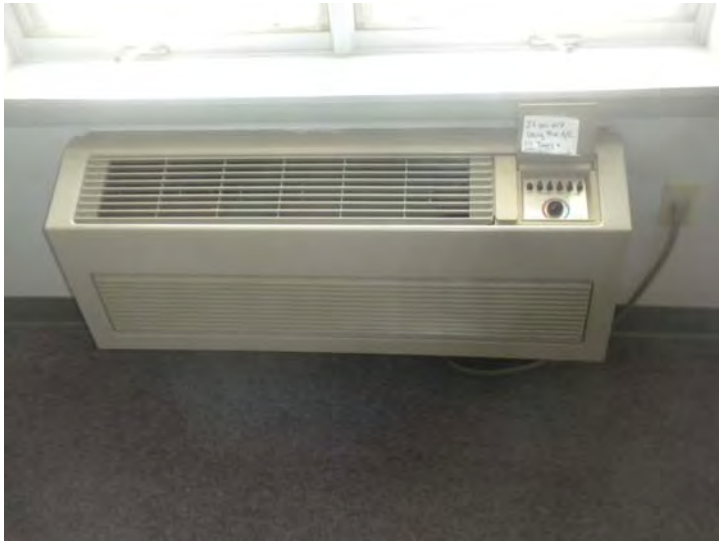
One of the thru-wall heat pump
