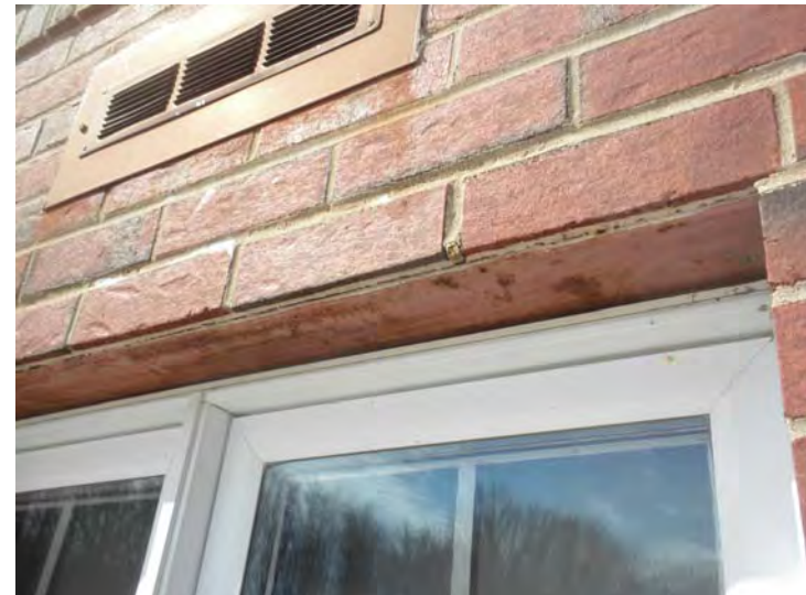
View of a rusted window lintel
