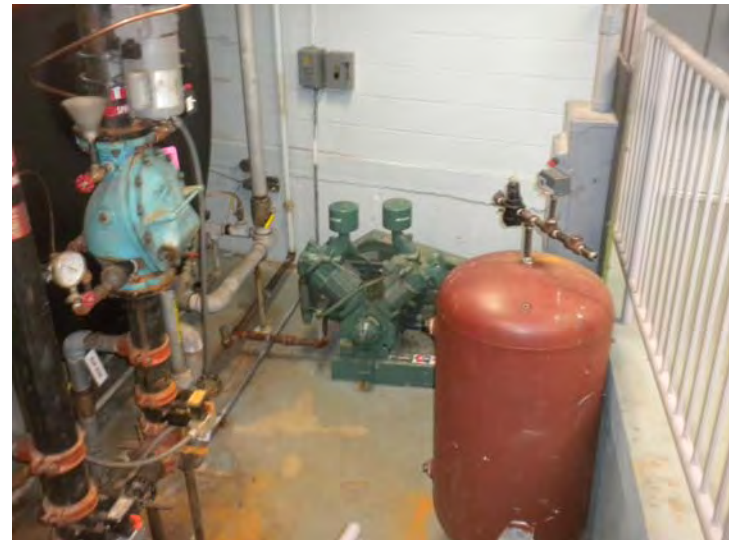
View of the fire suppression system compressor
