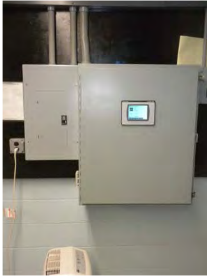
The well pump controls
