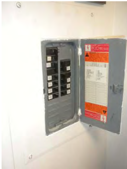
Dwelling units feature individual circuit breaker panels
